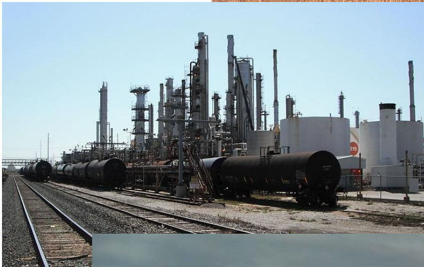
Oil refinery and railroad tanker cars
