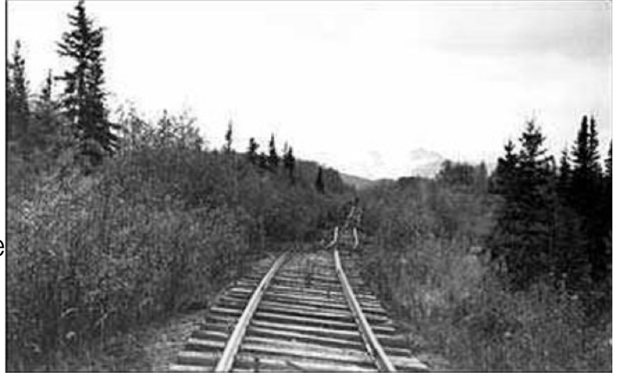
Old photo of a railroad in a place that has permafrost. Freezing water expands and pushes the rails out of line. Permafrost is ground that is always frozen below the surface. The top layer often thaws on warm days and then freezes again during cold nights.
