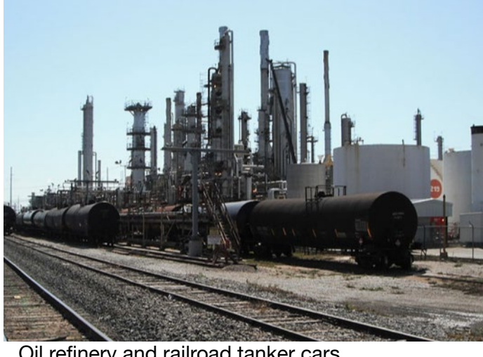
Oil refinery and railroad tanker cars
