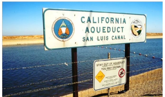
This “artificial river” is part of the California Aqueduct system. The system uses dams to block rivers in high mountains. These dams make reservoirs (man-made lakes) to store water from melting snow. Then artificial rivers (like this one) and huge pipes bring the water to the fields and cities of California.
